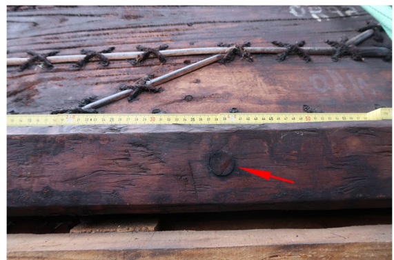
Fig. 15 Treenail fastening floor timber (FR 9) to the keel
