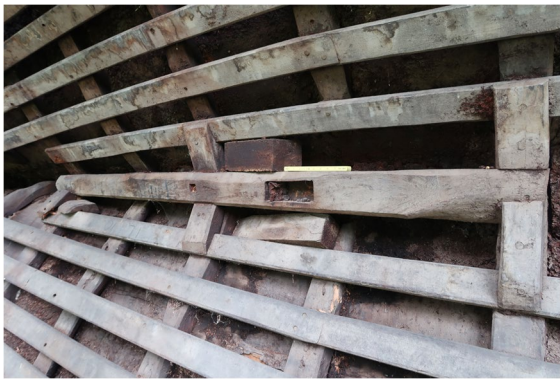
Fig. 22 Overview of the ceiling planks, mast step, and buttresses
