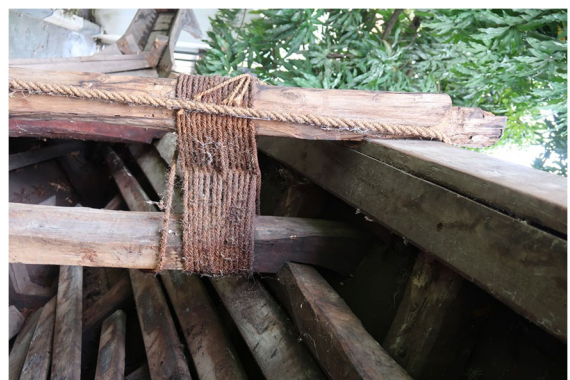
Fig. 23 A pair of forward through-beams lashed with coir rope. Note that the lower beam is notched over the shelf clamp while the upper beam is notched over the cap rail
