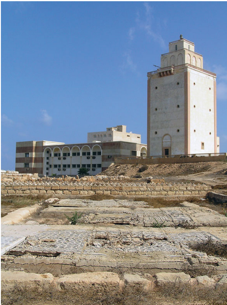
Fig. 10 An “exploded” mosaic caused by the use of salinated concrete for display, Sidi Khrebish, Benghazi (photograph by Paul Bennett)
