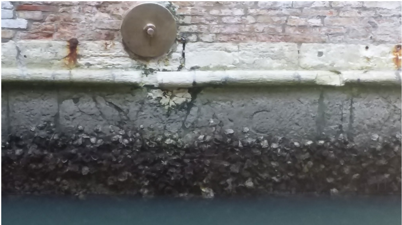
Fig. 1 One of the letters “C” with which the Venetians used to identify the Comun marin , i.e., the limit of the dark band of cyanobacteria which marks mean high-water level. The “C”, that was carved just on
