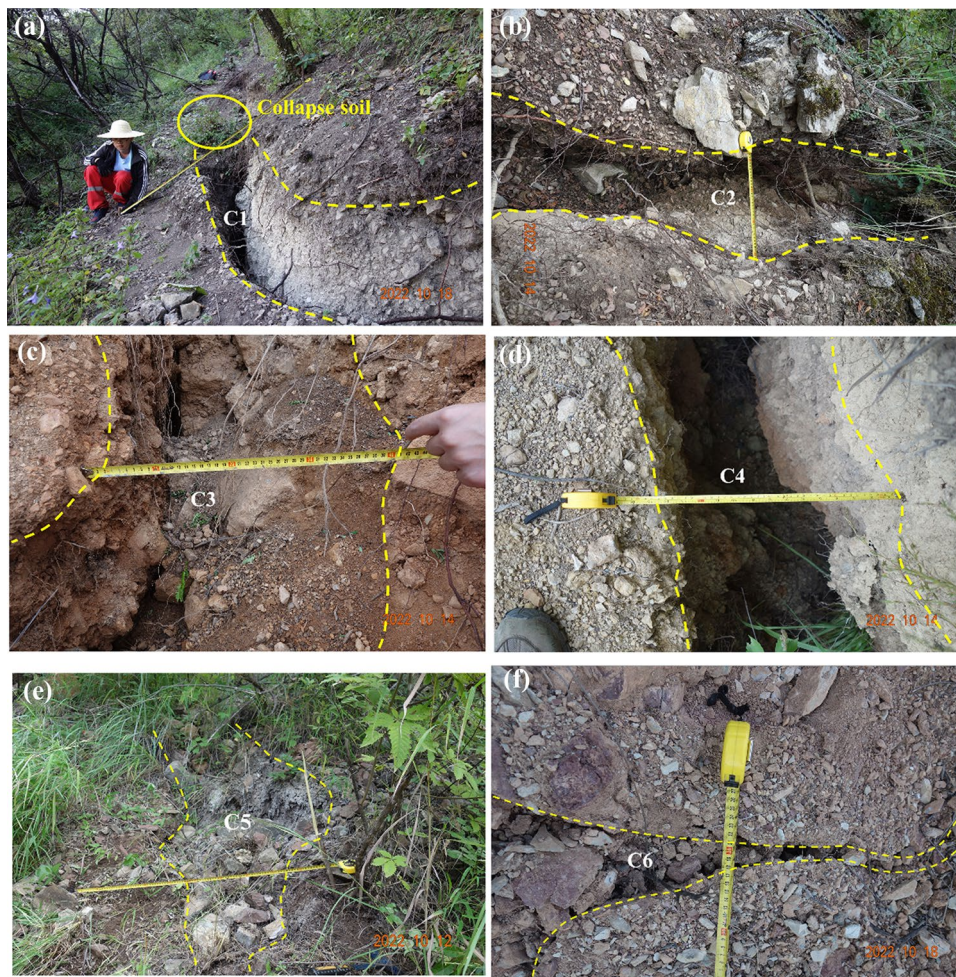
Fig. 5 Photos of typical cracks on the surface of the TDG landslide
