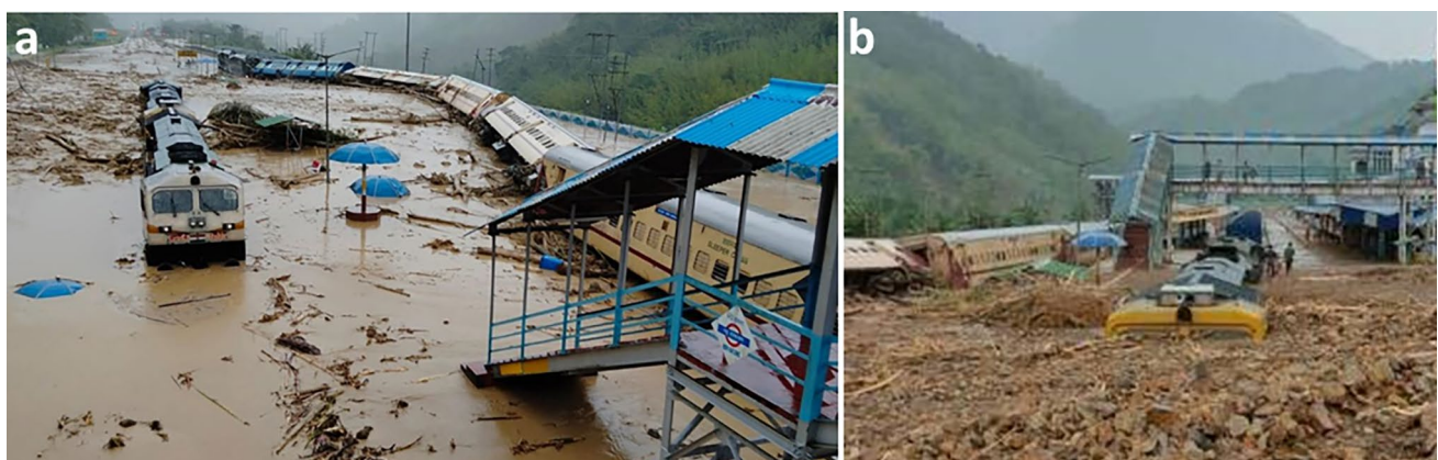
Fig. 2 a New Haf-long railway station covered with debris from landslides triggered around the adjacent slopes (source: www.downtoearth.org.in ). b Railway locomotive buried till roof under debris (source: www.indianexpress.com )
