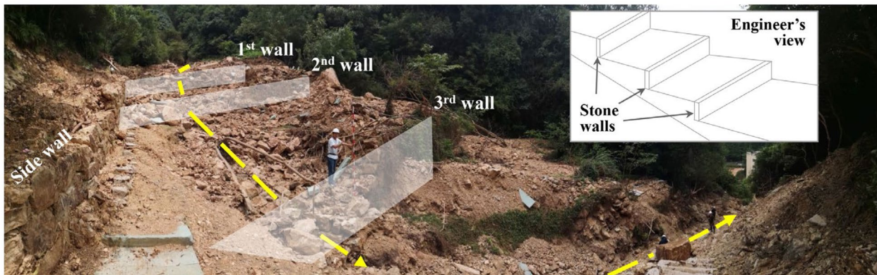
Fig. 22 Debris stone barrier walls behind the hotel
