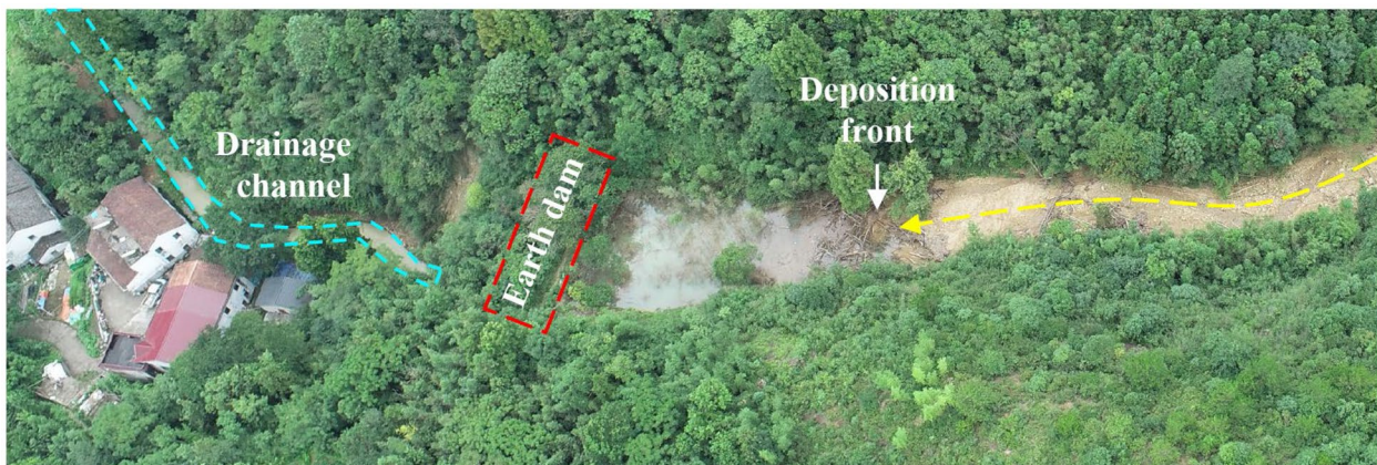
Fig. 23 Constructed earth dam behind the local village
