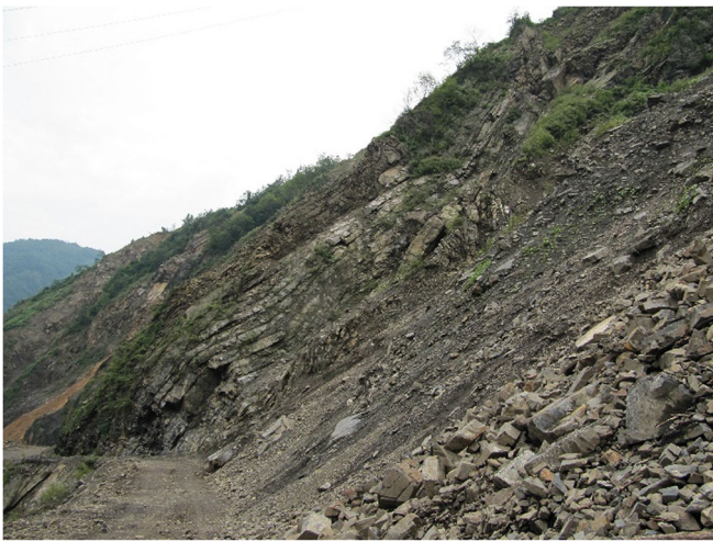
Fig. 17 Buckling failure triggered by Wenchuan earthquake (Qi et al. 2015)
