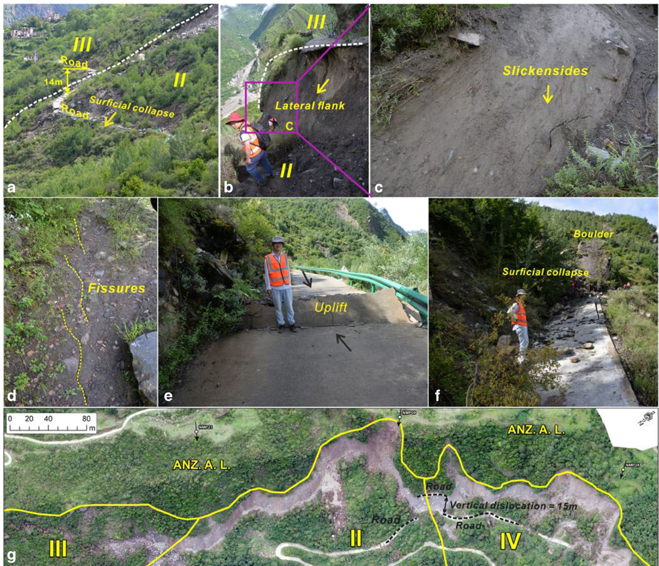
Fig. 12 Typical characteristics of main deformation zone II. (O) obvious dislocation in the local scarp area, (A and B) dislocation of a road and a lateral flank at the upstream boundary, (C) slickensides on the upstream flank, (D) numerous fissures at the downstream boundary, (E) uplift of a road in the middle section of zone II, and (F) a surficial collapse in zone II. The locations of (A), (B), (D), (E), and (F) are listed in Fig. 9
