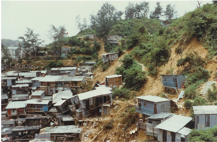
Fig. 10 Vulnerable squatter huts on sloping ground
