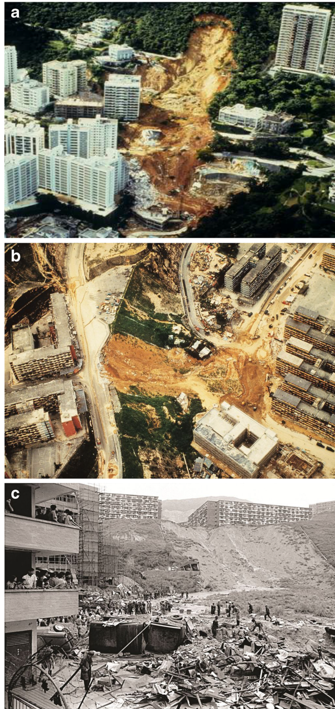
Fig. 3 The fatal landslides at Po Shan Road and Sau Mau Ping in the 1970s. a 1972 Po Shan landslide (a 12-storey building was completely destroyed and the top four storeys of an adjacent building were torn off, causing 67 fatalities). b 1972 Sau Mau Ping landslide (debris covered the resettlement area causing 71 fatalities). c 1976 Sau Mau Ping landslide (debris poured into lower floors of building causing 18 fatalities)
