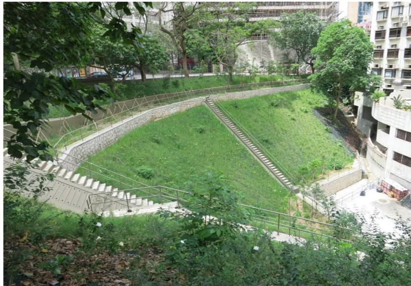
Fig. 7 Slopes retrofitted under the LPM programme with landscape treatment to enhance aesthetics
