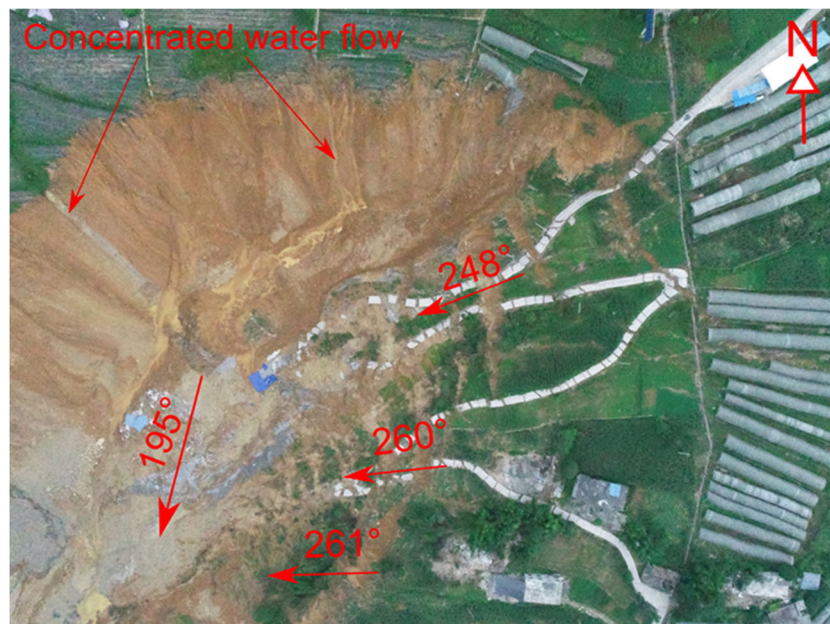
Fig. 4 Minor scarps at the head, showing the displacement of the sliding mass to the gully on the west side
