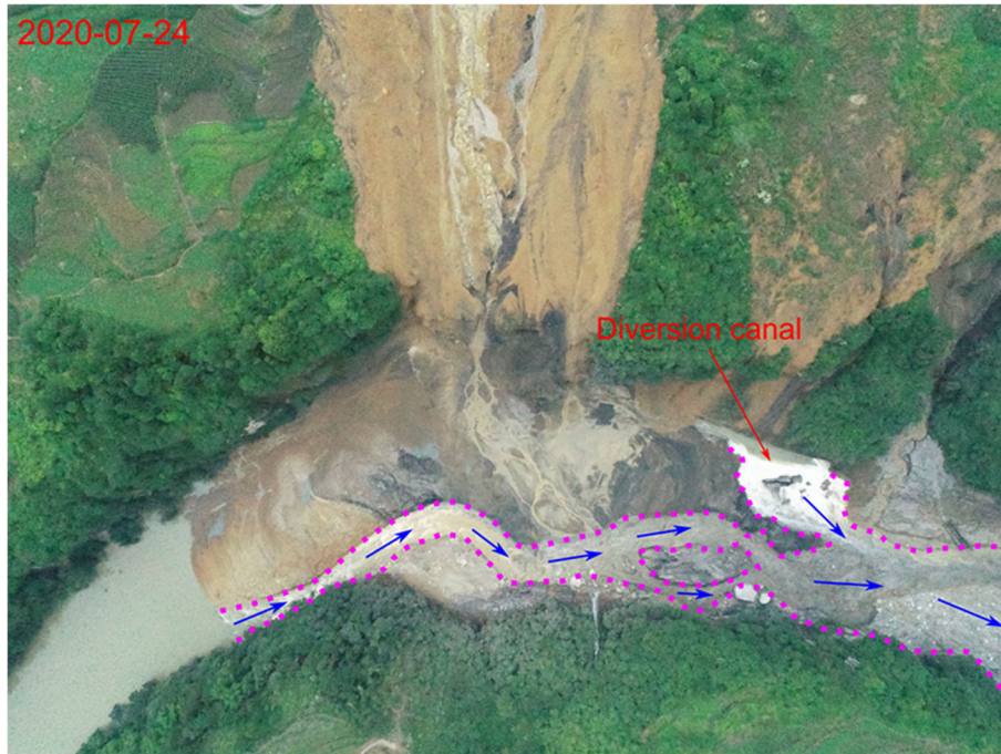
Fig. 5 Spillway formed on the top of the landslide dam
