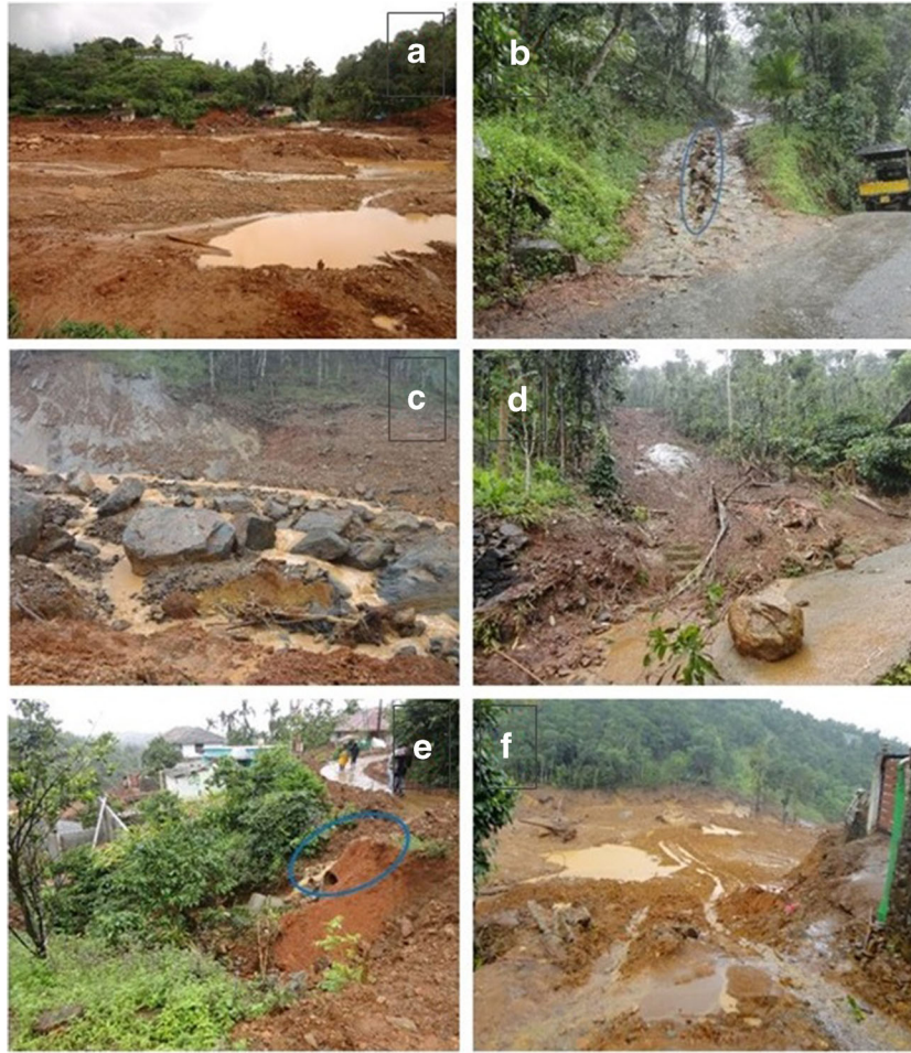
Fig. 8 The landslide and floods at Puthumala, Wayanad (site 2). a The damages due the flood in the tributary of the Chaliyar River. b Rain water draining downslope carved its own new consequent course along the leveled and stone paved path resulting in the caving-in or sinking of path in the middle. c Large boulder blocks of freshly cut rocks transported as rolling bed-load by floodwaters in the river. d One of the landslides at Puthumala, showing rolled boulder and exposed bedrock after stripped-off of its overlying weathered zone and soil cover. e Improper hill-side drainage of storm/rainwater and improperly placed culvert. f View from downslope of a landslide at Puthumala that washed away houses built within the channel course. Photo source: Authors
