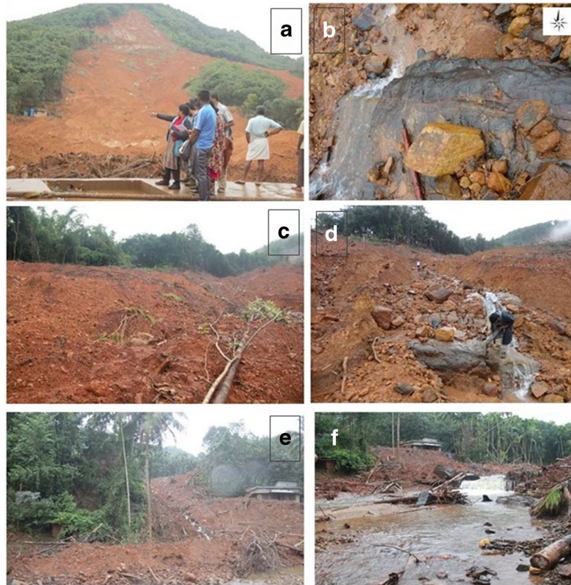
Fig. 4 Effects of landslides at site 1: Kavalappara. a Synoptic view of the major landslide. b Prominent dip-slope joints in the bedrock exposed after stripping away of overburden at Kavalappara major landslide. c Debris-covered run-out material at middle reaches to downslope. d Sediment-charged activated stream dislodging large boulders along the joints and resulted in formation of cascading rapids. e Western part of landslide where large blocks of rocks rolled down the slope. f Bank erosion and channel bed-load forming a channel bar, thus bifurcating the channel carved during the flooding of the Chaliyar River. (Photo source: author's personal collection at Amrita Vishwa Vidyapeetham, Kerala)
