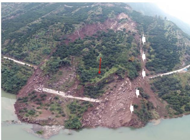
Fig. 17 The full-face photo of the Kamenziwan landslide. The white arrows indicate the position of the slide bed, suggesting that the landslide shear outlet is near 174 m
