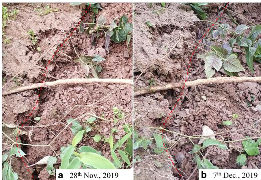
Fig. 4 The crack change in point E on November 28 (a) and December 7 (b). The crack was partially lowered by 5 cm on December 7
