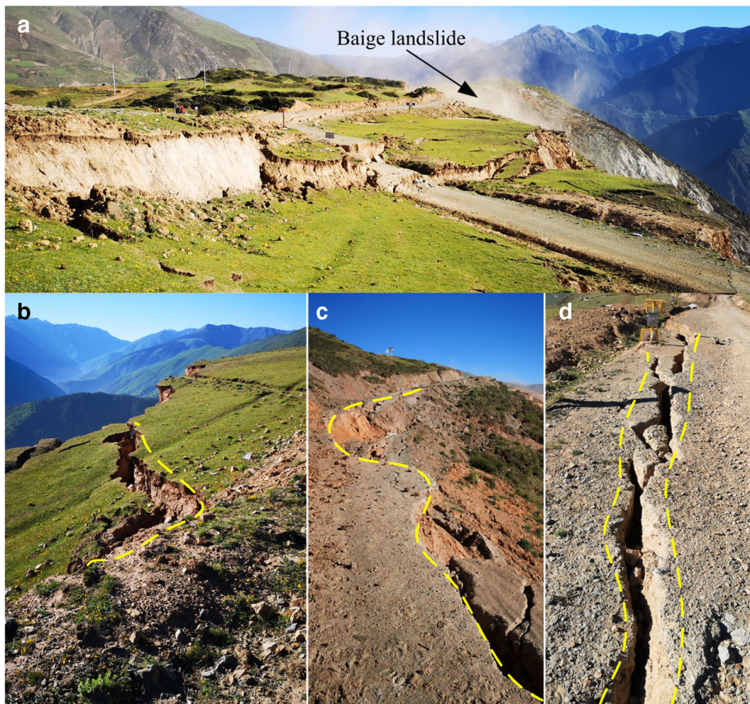
Fig. 12 Tensile cracks on the slope after the Baige landslide
