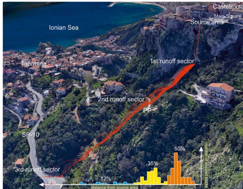
Fig. 4 2019 rockfall trajectory simulation with identification of the main runoff sectors
