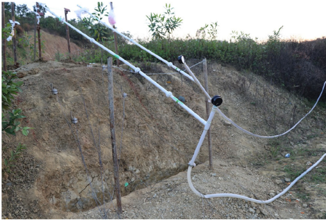
Fig. 5 The image of the testing slope in the field test
