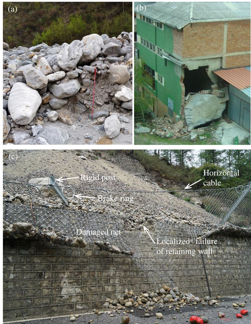
Fig. 1 a Debris flow deposition with granite boulders of varying diameters floating on the free surface in Tianmo Gully, Tibet, China. Alpenstock in the figure has a length of 1.2 m. b Localized punching failure of rigid wall by the impact of a 30\text{-m}^3 rock block in Santa Coloma, Principality of Andorra (Mavrouli and Corominas 2010). c Successful interception but failure of a rockfall flexible barrier under the impact of pebble flow, energy dissipating devices (brake rings) not triggered
