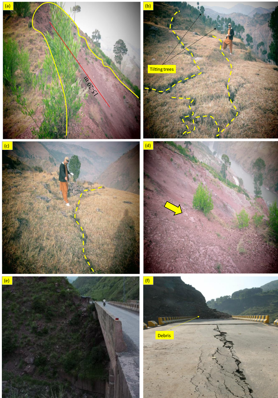
Fig. 4 a Photograph showing the landslide initiation. b Tension cracks on the crown. c Agricultural land. d Exposed sandstone on the right flank. e Donga Kass bridge before landsliding in 2006. f Blockage of Neelum road due to debris and damage of deck slab of Donga Kass bridge after landsliding
