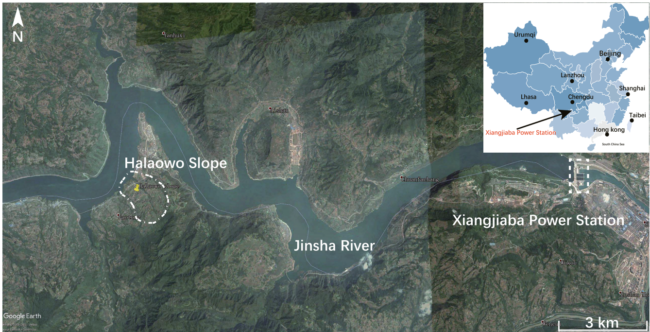
Fig. 12 The location of Xiangjiaba Hydropower Station and Halaowo Slope
