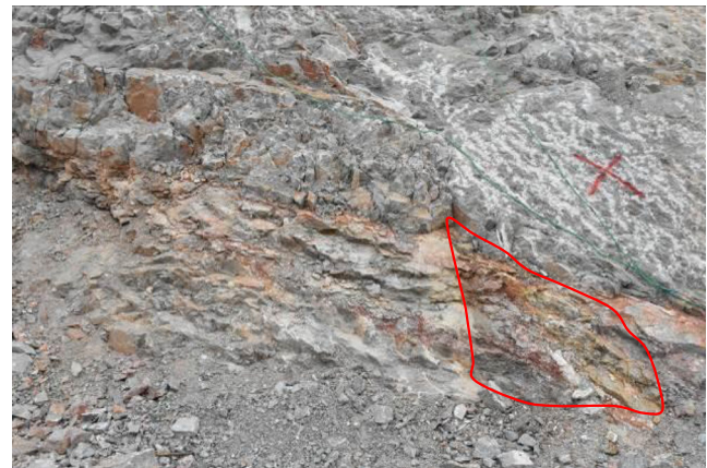
Fig. 5 Groundwater seepage at the foot of the slope
