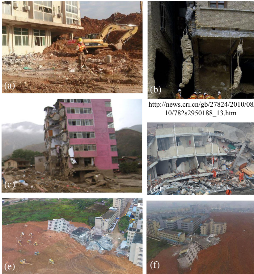
Fig. 6 Building damage states observed in Shenzhen landslide and Zhouqu debris flow
