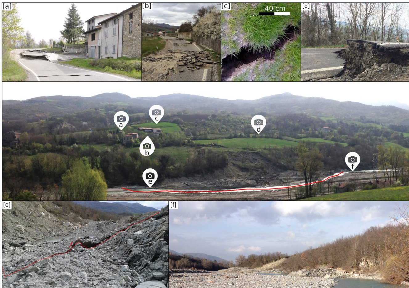
Fig. 2 Field evidences and damages to human infrastructures caused by the reactivation of March 2016: (a–d) evidences of movements occurred within the mobilized area and at its borders; (e, f) evidences of the streambed uplift
