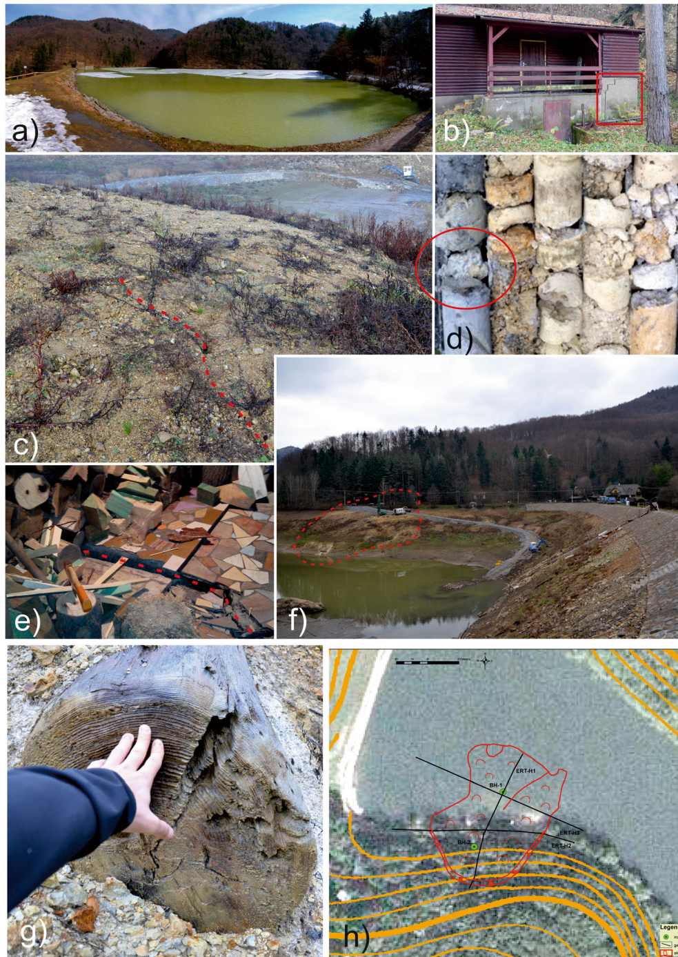
Fig. 4 Photodocumentation on active slope deformation. a General overview of Lower Hodruša mining water reservoir taken from the dam. b Detail photo of open cracks on one of the chalets situated in main scarp area. c Open cracks in accumulation part of the active landslide. d Material of shear plane. e Open cracks inside of chalet. f Photo of active slope deformation taken from the dam. g Old remediation works from the eighteenth century—oak wood posts. h Situation map of landslide with realised boreholes and geophysical measurements profiles
