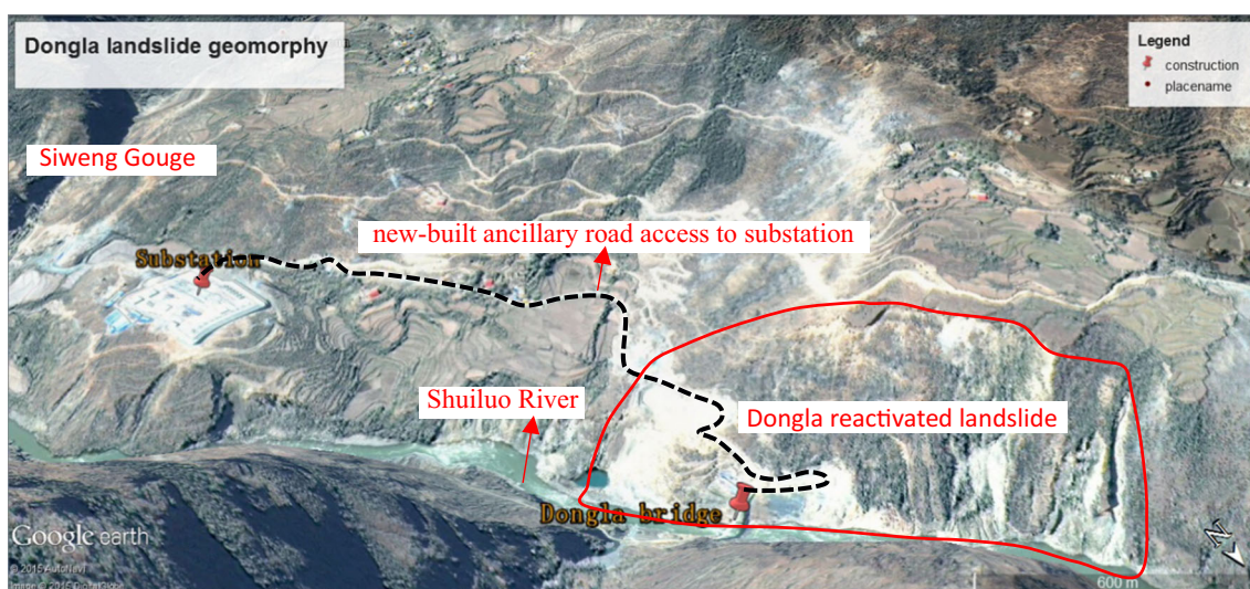
Fig. 3 Location of the Dongla Bridge and Dongla Reactivated Landslide. The construction of the Dongla Bridge and the new ancillary road (black line), as well as the gold mining pits and the gold washing pond destabilized the slope
