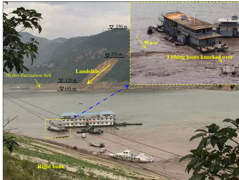
Fig. 2 Photos of the Hongyanzi landslide site, showing fishing boats damaged by the landslide-generated wave
