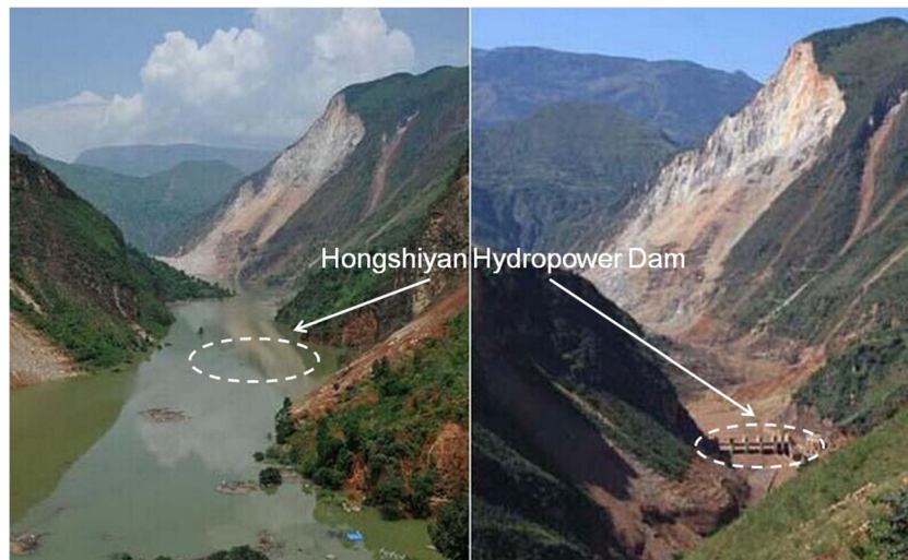
Fig. 9 The landslide lake before and after drainage (based on QQ News 2014)
