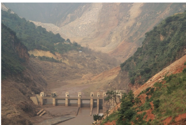
Fig. 12 Water impounded in the dammed lake has been released by the new constructed channel. As shown in this picture taken on October 10th, the submerged artificial concrete dam has been exposed
