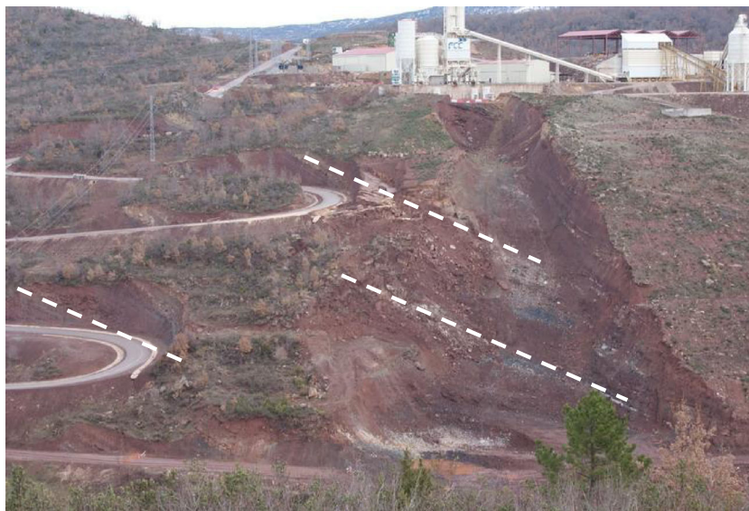
Fig. 19 Planar failure in Castrovido claystone controlled by sedimentation planes
