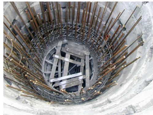
Fig. 11 Interior of the shaft during the execution of the secondary lining
