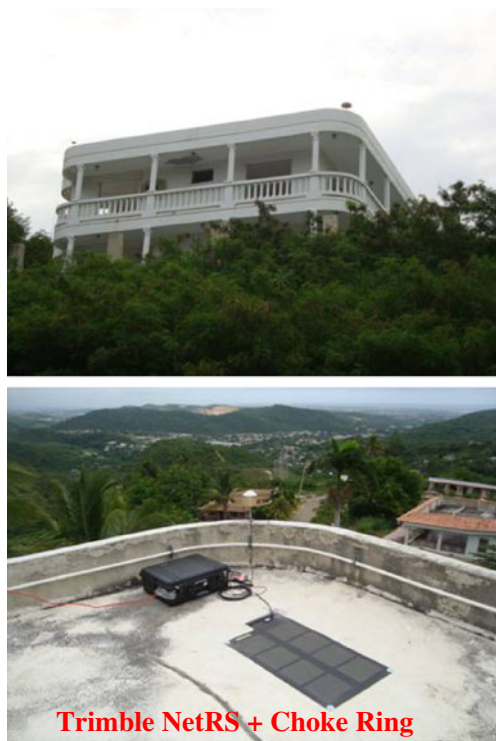
Fig. 10 The continuous GPS station on the two story building at the head of the landslide. The GPS station was equipped with a Trimble NetRS GPS receiver and a choke ring antenna. The GPS receiver was powered by a battery charged by solar power
