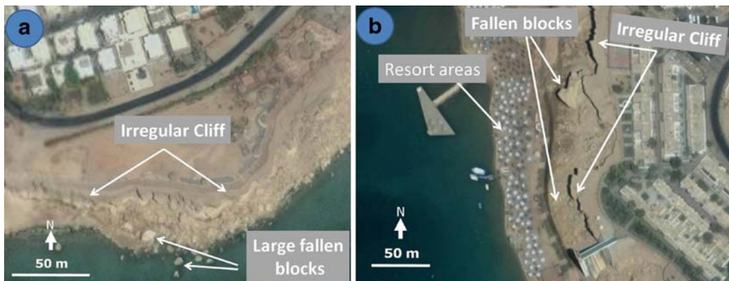
Fig. 3 High-resolution image (QuickBird acquired on June 2nd, 2007 with 61 cm spatial resolution) showing a portion of cliff in the study area. a The presence of large boulders under the irregular cliff. b The distribution of resort areas under an
