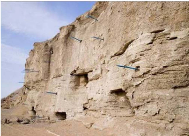
Fig. 19 Distribution of anchor cables outside the cliff surface before cutting off
