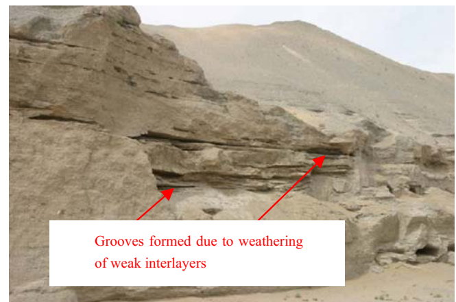
Fig. 13 Weak interlayer in the north area
