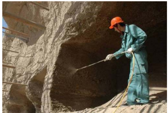
Fig. 22 Construction site of the weather-proof consolidation by PS spray
