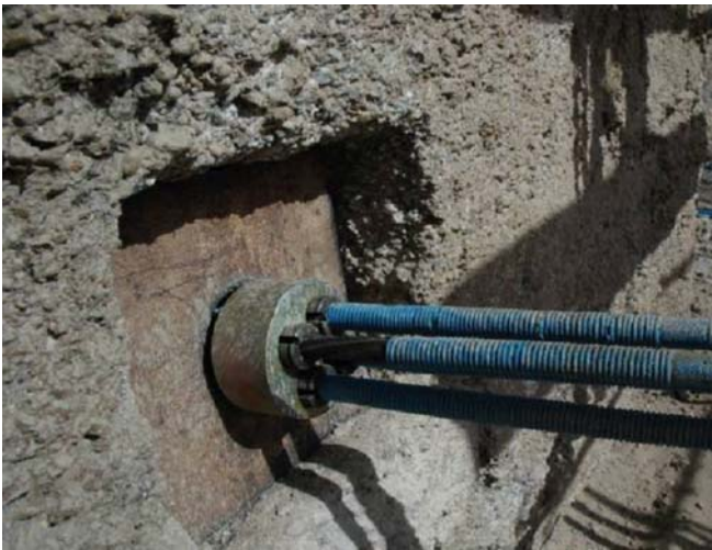
Fig. 18 Installation of an anchor plate
