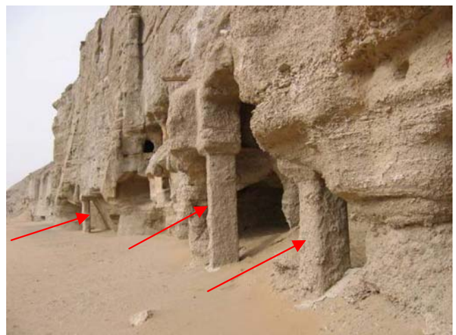
Fig. 23 Column support of the hanging sections at cliff bottom
