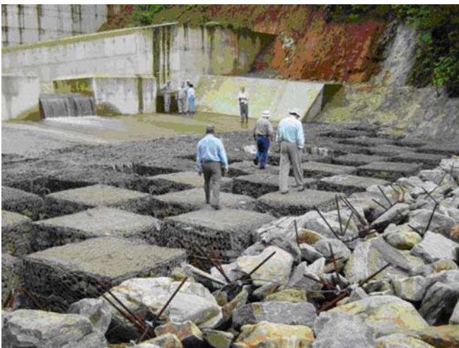
Fig. 23 Flexible mantle of reinforced gabions
