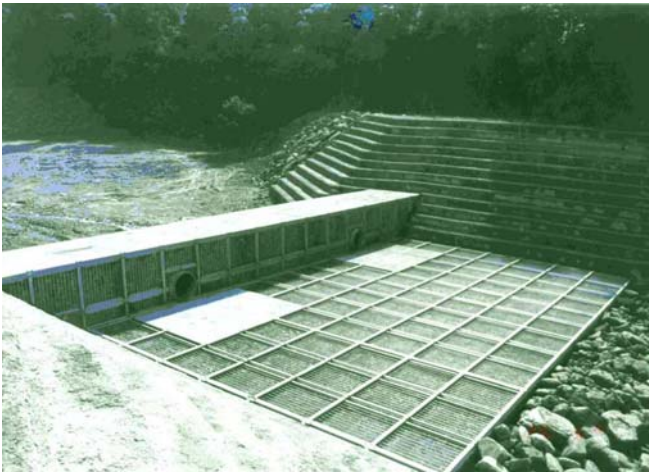
Fig. 22 Downstream view of a steel frame type dam (BS-1)
