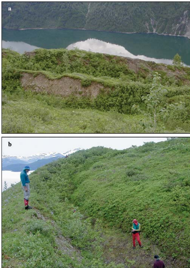
Fig. 6 a Uphill-facing rotational escarpments and resulting trough, roughly perpendicular to the downslope direction. b Relief at one of the escarpments. Direction of landslide movement is to the left (south)
