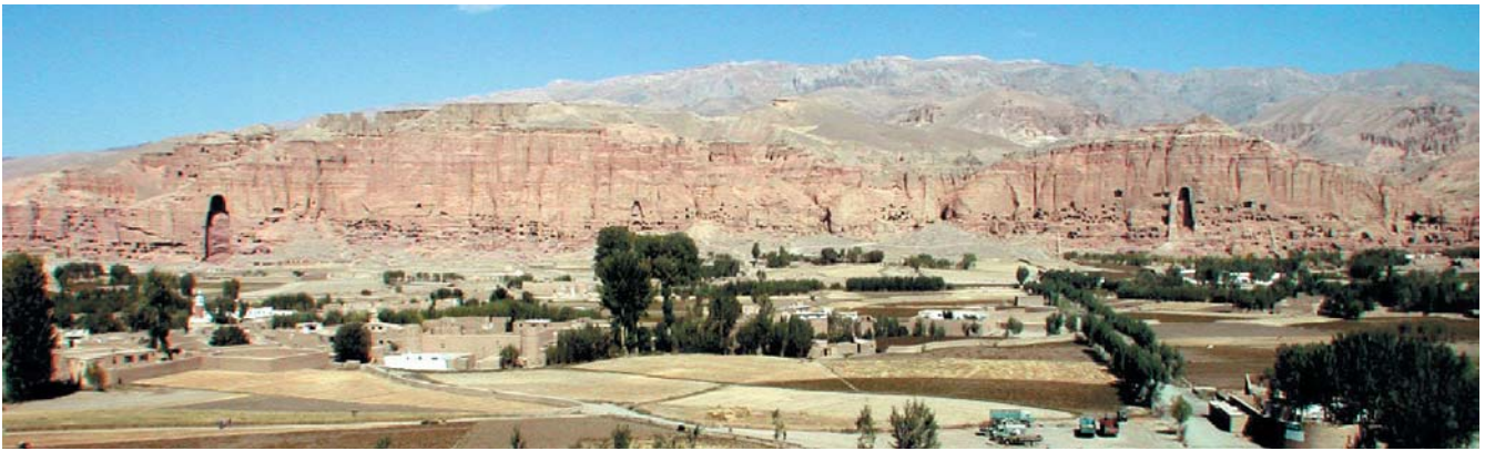
Fig. 2 View of the cliff at Bamiyan, central Afghanistan showing the relationship between the two Buddhas and the caves. The Great Buddha is on the left while small Buddha is on the right
