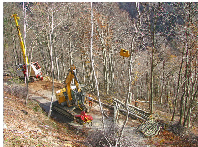
Fig. 2 Typical configuration of a cable yarding operation (site 4, WT)
