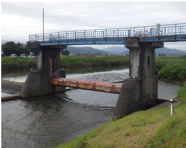
(a) Overview of monitoring structure.
