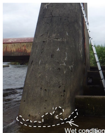
(a) The bottom part of the weir in the wet condition.
