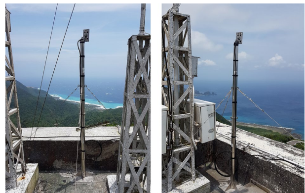
Fig. 2 GPS-R receiving antenna installations and views to the sea from the Lanyu-ENE (right panel) and Lanyu-SW (left panel) systems
