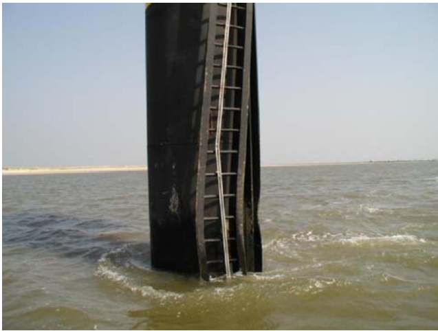
Fig. 4 Damaged external ladder of the time-series station after a commercial fisherman's boat had run into it in May 2003
