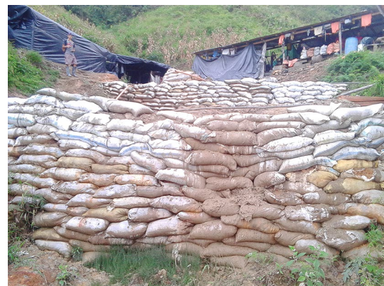
Fig. 3 Tailings sacks stacked as tailings repository in Virgen del Carmen ASGM site in Santa Inés
