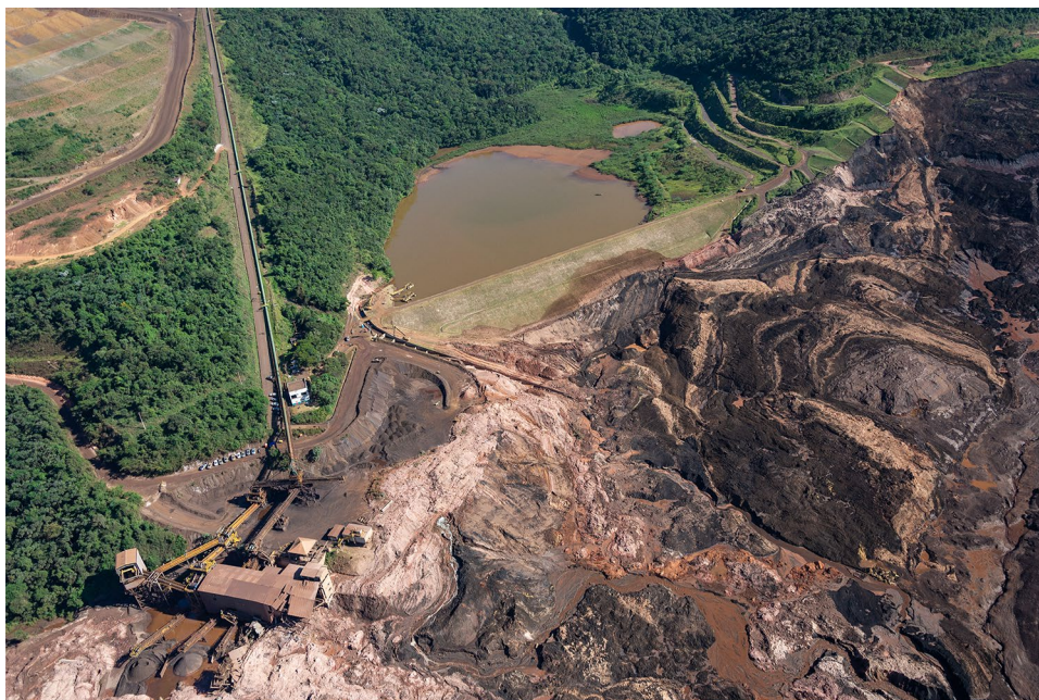
Fig. 1 Brumadinho tailings storage facility after dam failure. Source: Vinicius Mendonça/Ibama, under cc-by-sa-2.0 license, https://creativecommons.org/licenses/by-sa/2.0/deed.en
