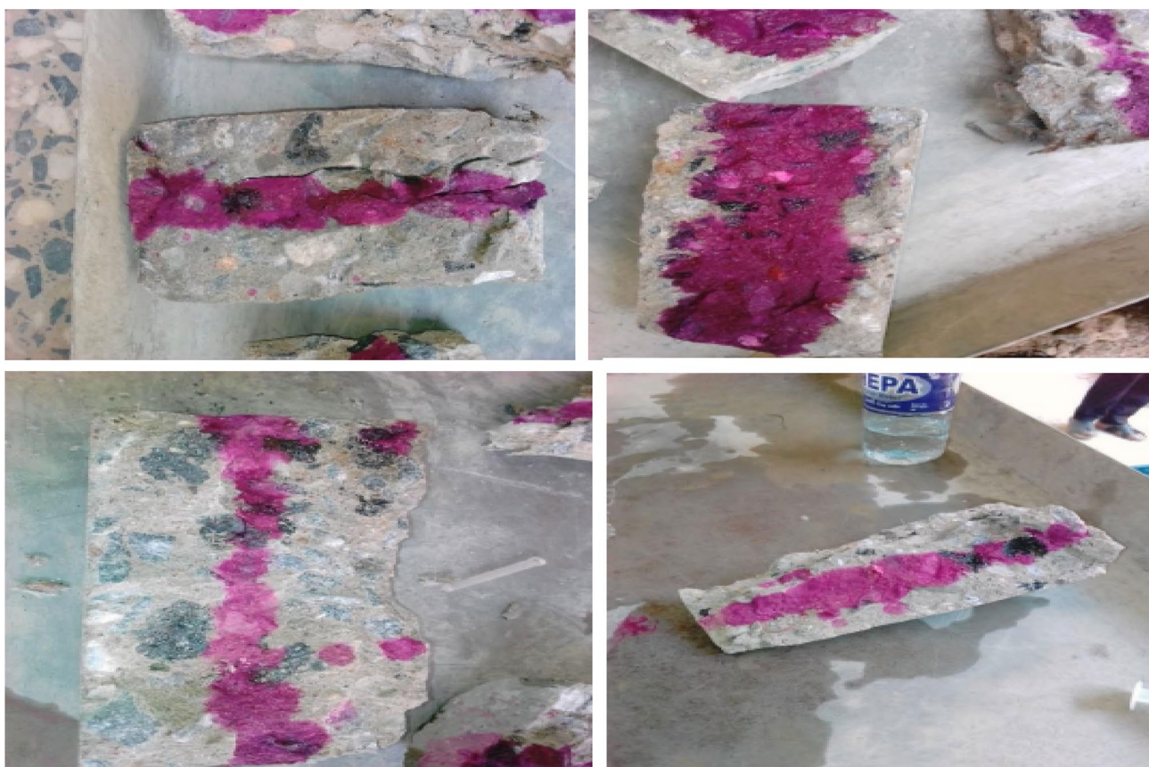
Fig. 2 Carbonation depth of concrete using phenolphthalein and ethanol
