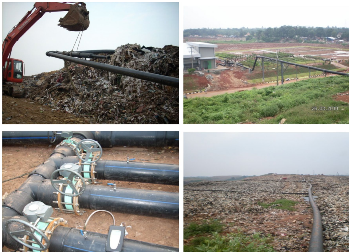
Fig. 6 Pipeline installation and gas collection at Bantar Gebang Landfill—Bekasi (authors' collections)
