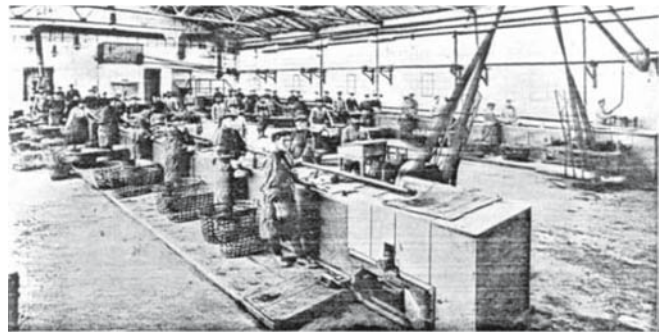
Fig. 4. Sorting plant in Munich-Puchheim (1907)
