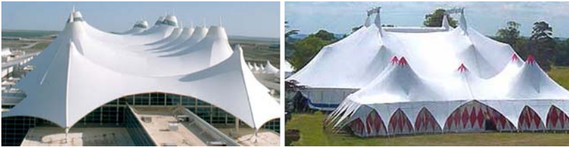
Fig. 2 Roof of the Denver International Airport and protrusions in a big top tent
