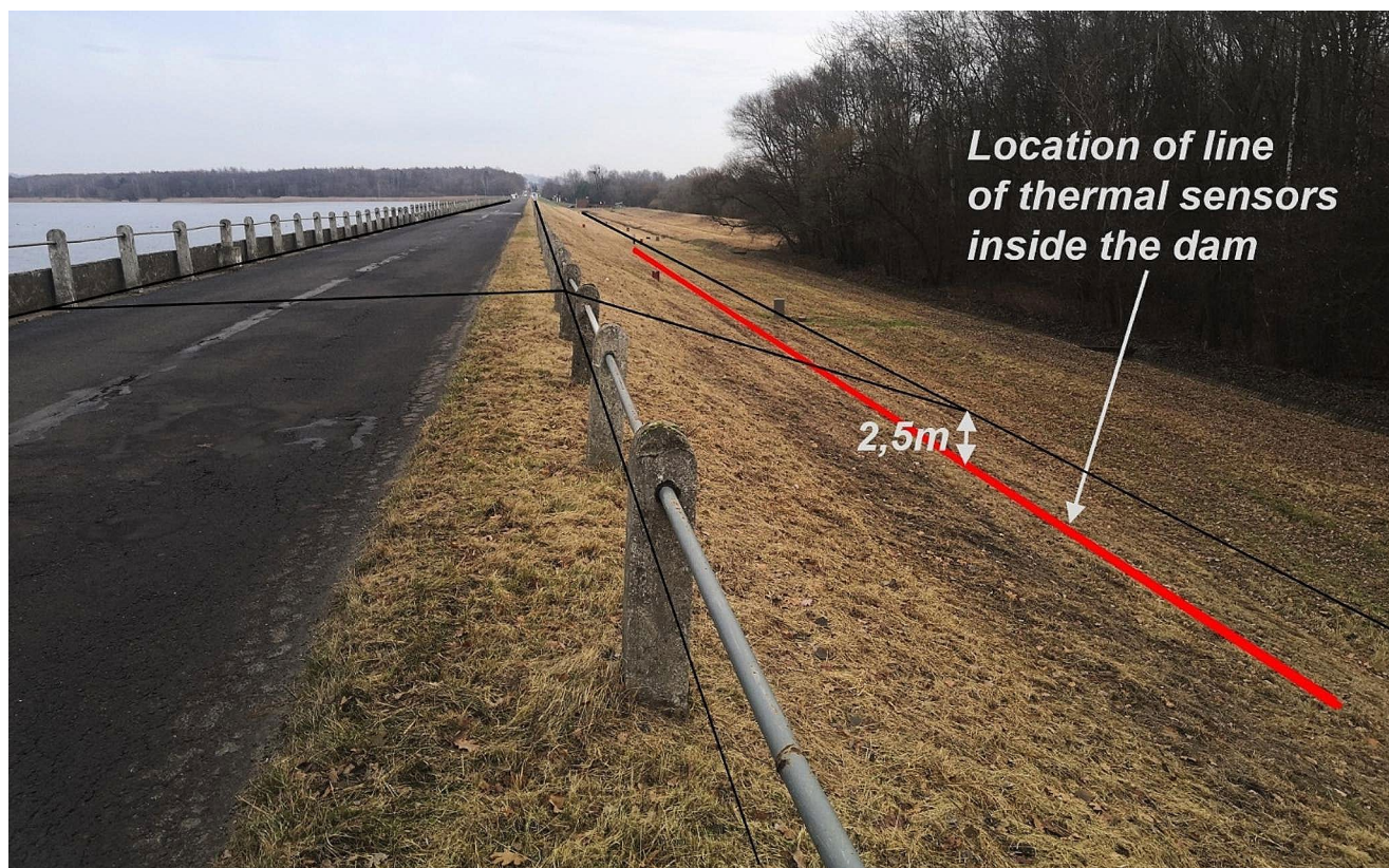
Fig. 8 Crest and land-side part of the Kozłowa Góra dam including location of thermal sensors in its landside toe
