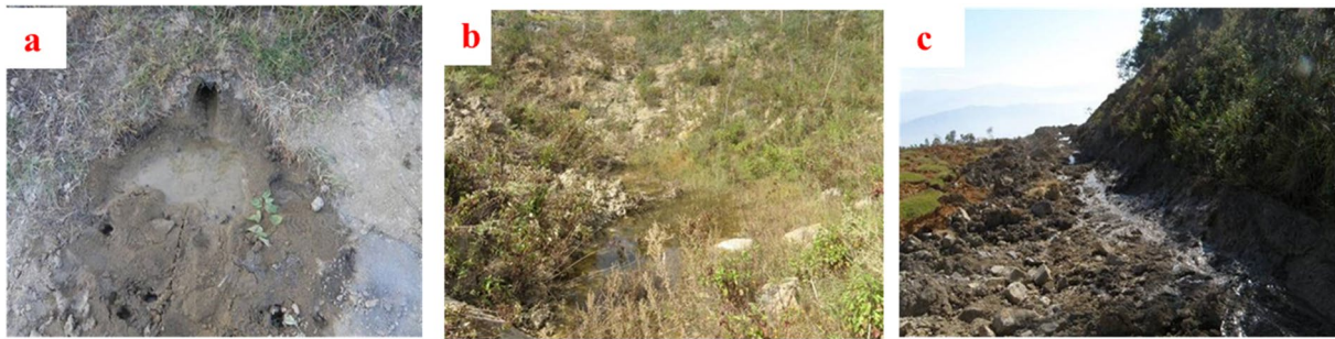
Fig. 10 Surface water exposures observed in the landslide area during field investigations (the approximate locations are shown in Fig. 6a). a Groundwater outflow from part drainage holes seated in the filled
