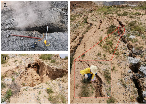
Fig. 1 Photographs of surface collapses that have occurred in the coal fire control project site after grouting/watering was used to extinguish coal fires in Shaanxi Province, China, showing the following: a single crack; b surface subsidence; and c crack zone
