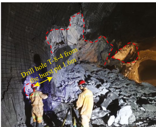
Fig. 5 Boreholes T-8-2, T-8-3, and T-8-4 around the rockburst pit
