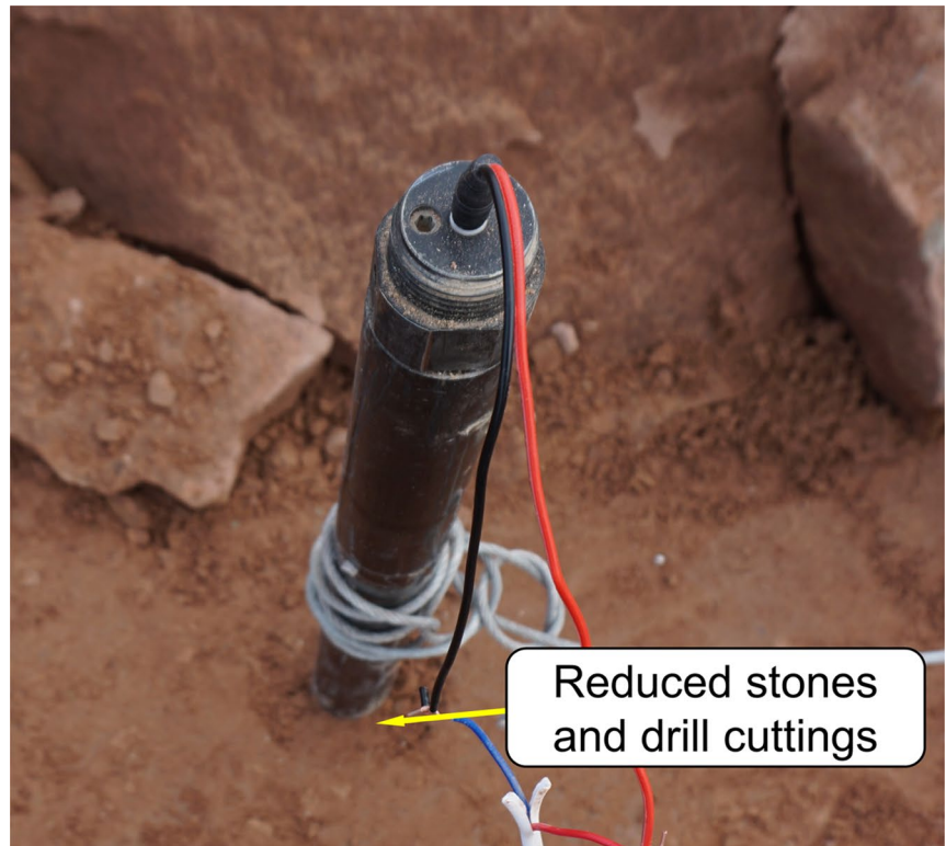
(a) Stemming with reduced stones and drill cuttings
