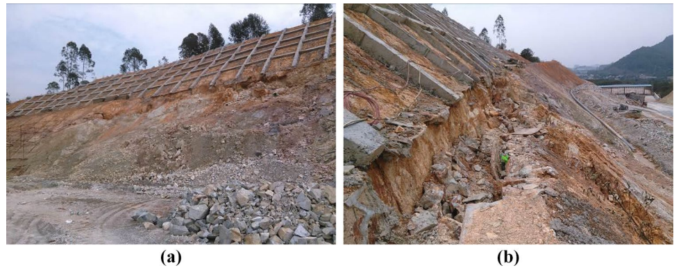
Fig. 6 Status of the slide after the modified excavation in January 2016
